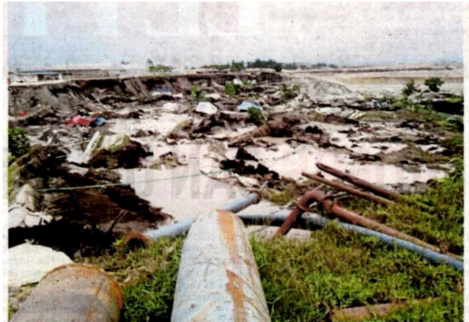
The land subsidence that struck an area near Jalan PKPS in Kampung Bestari Jaya, Kuala Selangor, on Friday. PIC COURTESY OF THE FIRE AND RESCUE DEPARTMENT
